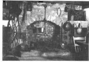
Old fireplace in slave quarters section of Fur Trading Post. Note keystone arch in fireplace.
