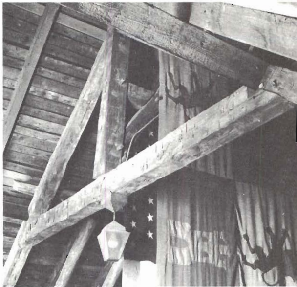
Great oak beams of Guibourd-Valle Norman truss are pegged in place.
