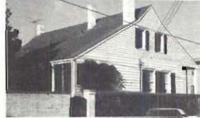
Rear gallery of Guibourd-Vallé house has been glassed in with casement windows, overlooks one of Ste. Genevieve's most handsome gardens.
