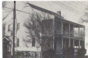
Bolduc-LeMeilleur House before restoration.
