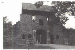
Main gate at Fort de Chartres has been restored. Structure holds cannon platform.
