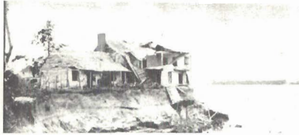
Photo taken during flood of 1881 shows Mississippi swirling about old Kaskaskia house.
