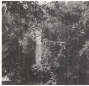
View from bridge over Saline in Perry county shows power of forest to conceal the Burnt Mill.
