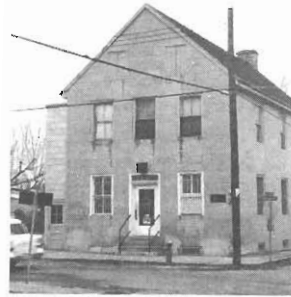
The Dufour-Rozier Building
