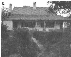
Rear of Bolduc from orchard shows old boxwoods in formal garden, brick kitchen under gallery at left.
